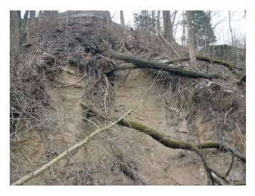
**Photograph 11**: Upper slope failure in Area 4 below 14 Mile Road Appendix A List of Figures/Photographs
