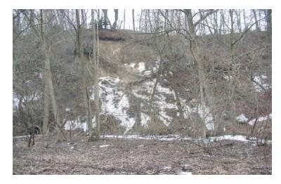
**Photograph 7**: Upper slope failure in Area 3 along 14 Mile Road
