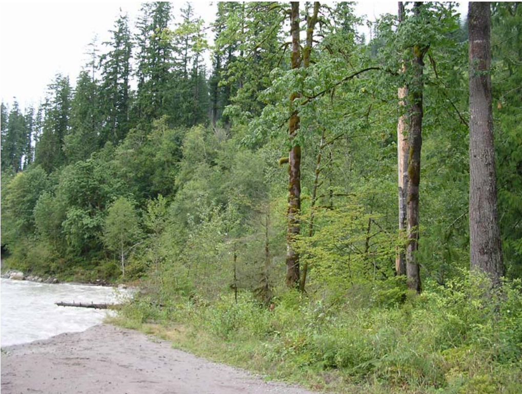
Photo 2. View from upstream end of washout looking downstream.
