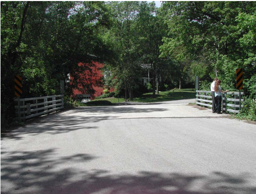
Williamsburg Bridge #2, from the east
