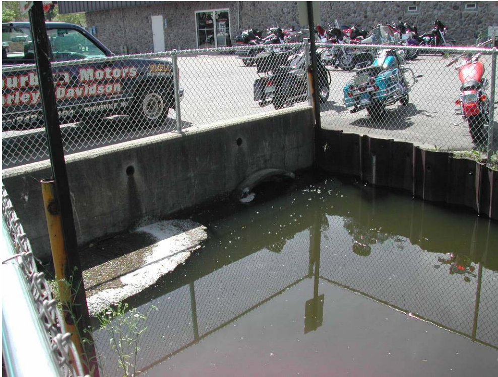
Car lot culvert outlet, west edge of Harley Davidson lot
