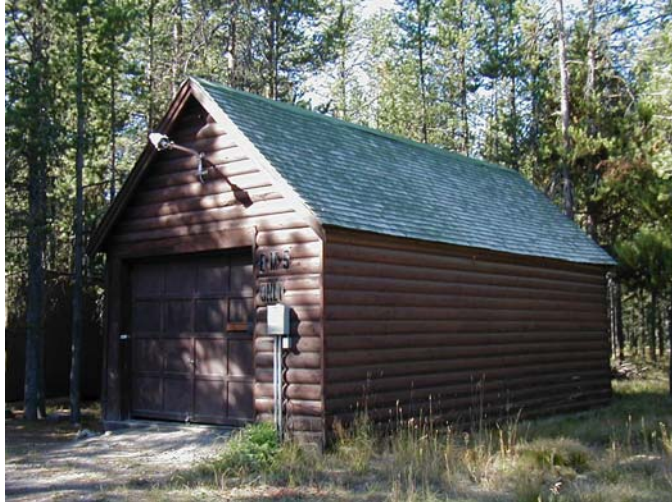
Photo: Flat Rock Garage
