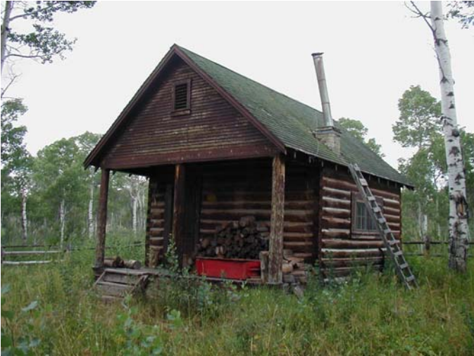
Photo: Brockman Guard Station Cabin
