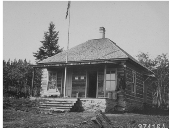
Grandview Ranger Station, 1918
