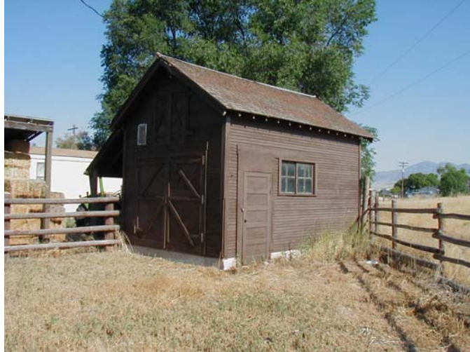
Photo: Malad Warehouse Barn
