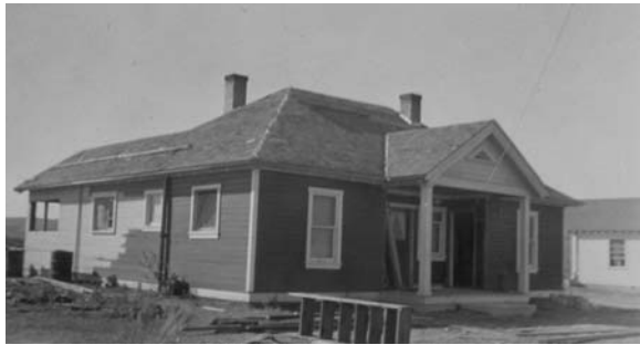
Swan Valley Ranger Station Dwelling, c.1934
