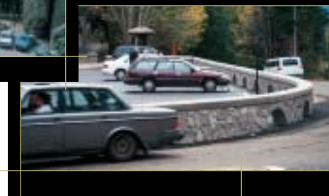
In an area of limited space, this parking lot is separated from the roadway by a low stone wall that mimics the design of historic walls along the byway. Historic Columbia River Highway, OR
