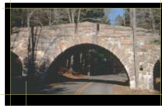
This bridge has additional arches on either side of the road, which gives it a lighter appearance and allows motorists to view more of the scenery. Acadia, ME
