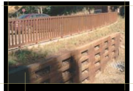
Timber crib walls are appropriate in rustic settings. San Juan National Forest, CO
