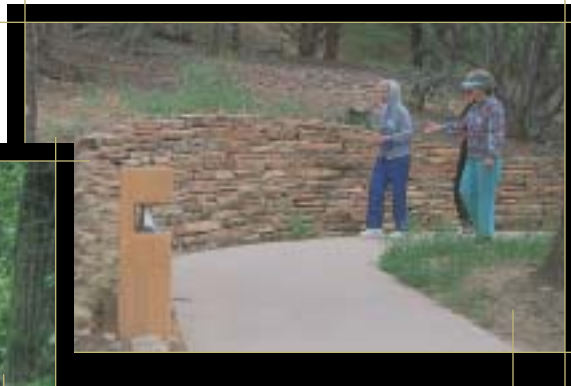
This native dry-laid stone retaining wall with its irregular height makes an attractive transition from the natural landscape to the paved trail with lighting. Ridgway State Park, CO
