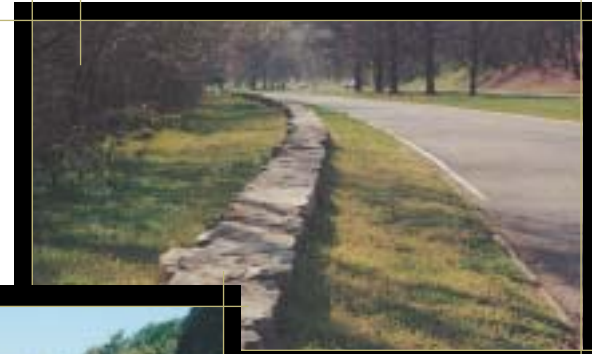
Stone walls can be used instead of guardrails to blend with other structures along the byway. George Washington Memorial Parkway, VA
