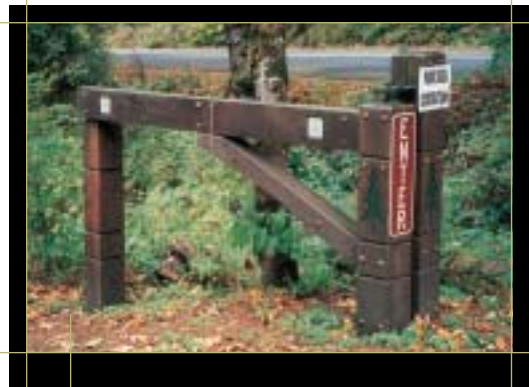
Bolts and scoring add nice details to this gate. Historic Columbia River Highway, OR
