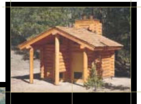
Vault toilets are widely used in semiprimitive settings where potable water is not available. Bridger-Teton National Forest, WY
