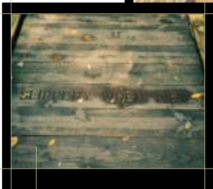
Although unobtrusive, this routed message warns visitors of a potential hazard. Highland Scenic Highway, WV
