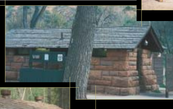
Flush toilets accommodate the high use at this site. The architectural style, building materials, and location all integrate it into the surroundings. Zion National Park, UT
