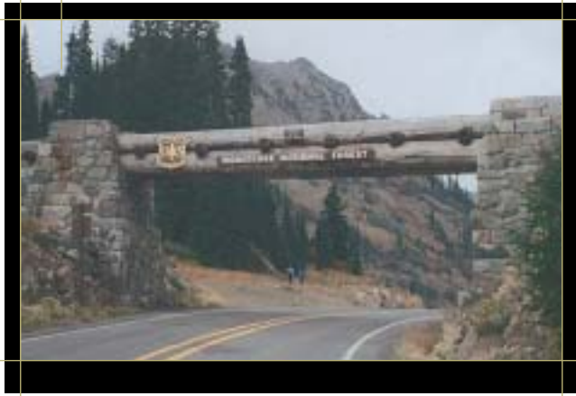
Stone columns and heavy log beams form a gateway. Mather Memorial Parkway, WA
