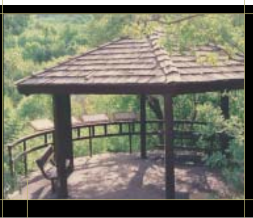
A roof structure extends the seasonal use of this overlook. Uinta National Forest, UT
