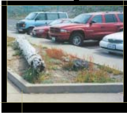
To integrate the parking lot into the surrounding terrain, logs and rocks from the eruption of Mount St. Helens were incorporated into planting islands, and native plants were allowed to regenerate. Spirit Lake Memorial Highway, WA
