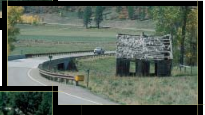
The horizontal alignment on West Delores Road curves around a historic structure to preserve it. San Juan National Forest, CO
