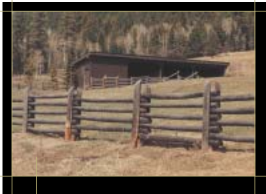
This double post-and-rail fence fits well into its setting. Upper San Juan River Valley, CO
