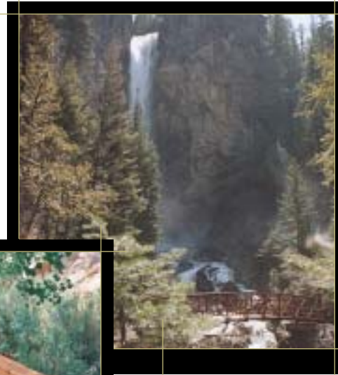
To safely transport visitors across a steep ravine, a naturally weathering steel bridge was installed that blends into the forested environment. San Juan National Forest, CO
