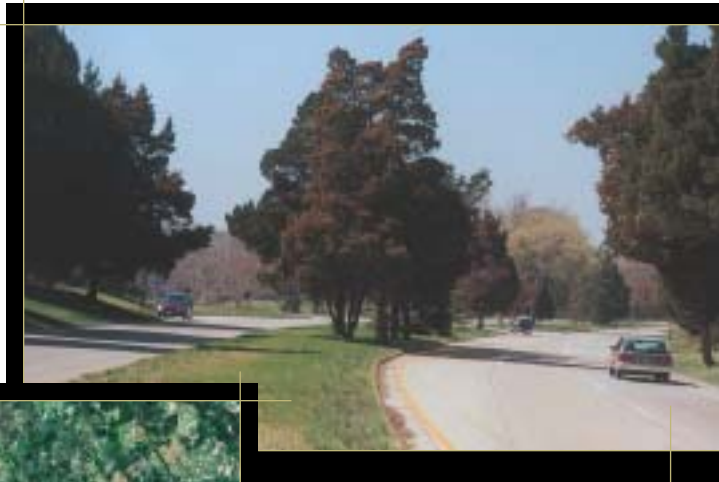
Trees and shrubs were planted in this median to visually separate the lanes of traffic and to blend the road corridor into the existing landscape. George Washington Memorial Parkway, VA
