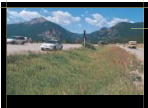
To reduce pollutants from entering natural waterways near Dillon Reservoir, road runoff is directed into grass-lined bioswales that collect oils and heavy metals. Interstate 70, CO
