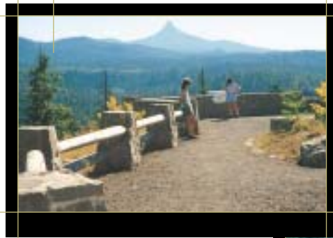
In the rugged Cascades, this overlook uses native stone and wood to define pedestrian areas and to protect visitors from the steep drop-off. McKenzie Pass–Santiam Pass National Scenic Byway, OR
