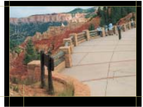
The color of the surrounding hills and spires are repeated in the stonework at this overlook. The long length of the railing allows large numbers of people to view at the same time. Bryce Canyon National Park, UT
