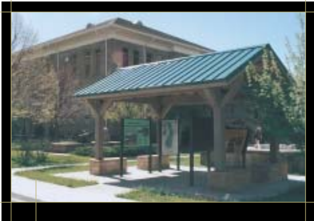
This kiosk complements the historic structure behind it, while providing an inviting place for visitors to receive orientation to the byway. The Energy Loop: Huntington & Eccles Canyons Scenic Byways, UT
