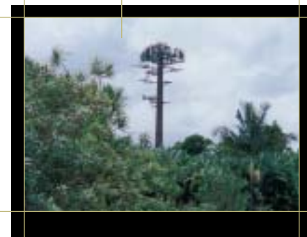
A microwave tower shaped like a tree blends into the forest ridge. Kauai, HI
