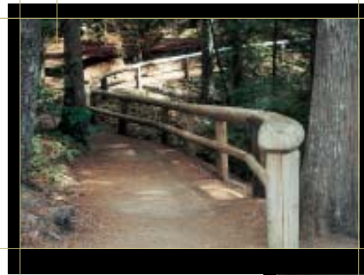
A curved branch was used as the terminus of this railing. It was shaped and sanded to fit the hand. McKenzie Pass-Santiam Pass National Scenic Byway, OR
