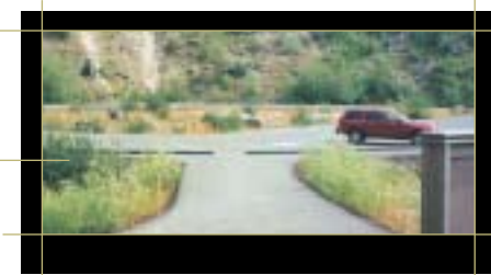
A biofiltration pond was incorporated into the design of this parking lot and planted with native plants. Spirit Lake Memorial Highway, WA
