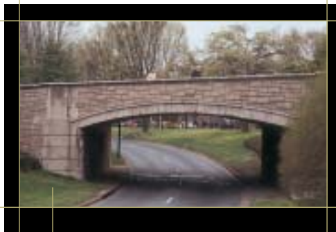
Use of native rock and concrete is combined to provide a highly attractive bridge. George Washington Memorial Parkway, Washington, DC
