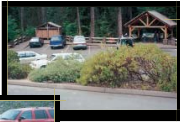
This parking area at Sahalie Falls is situated at different levels to fit the terrain. The planted areas help integrate it into the site.
