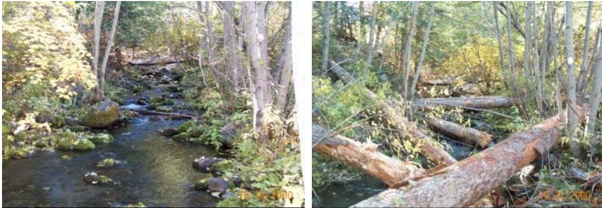
Figure 2. The photos above illustrate one work site in Ramsey Creek before and after log placement. Logs placed in the stream channel improve fish habitat and increase the number of times high stream flows spill over the banks onto the floodplain, thus improving riparian area health.
