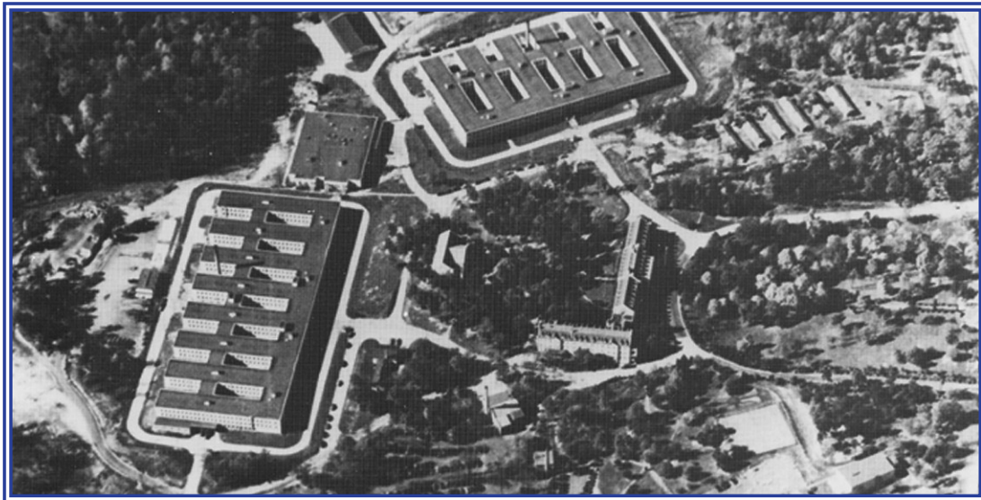
Aerial view of Arlington Hall Station
