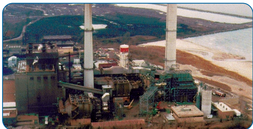
Pure Air's scrubber at Bailly Generating Station
