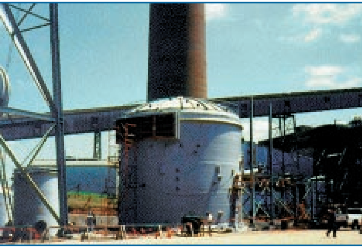
Chiyoda CT-121 Jet Bubbling Reactor constructed on-site using fiberglass-reinforced-plastic
