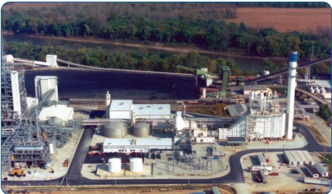
Wabash River Generating Station 262-MWe IGCC
