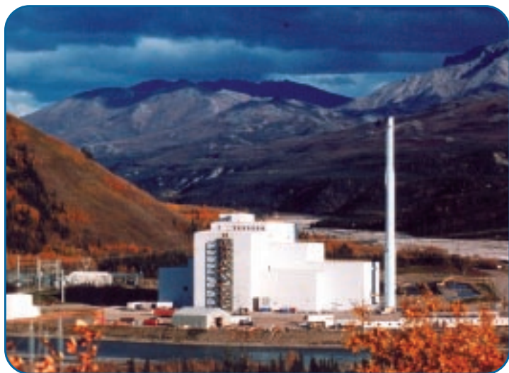
Healy Generating Station
