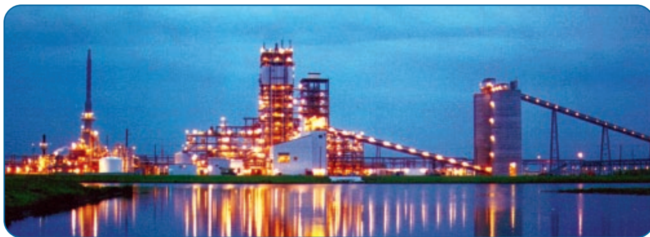
Polk Power Station 250-MWe IGCC facility
