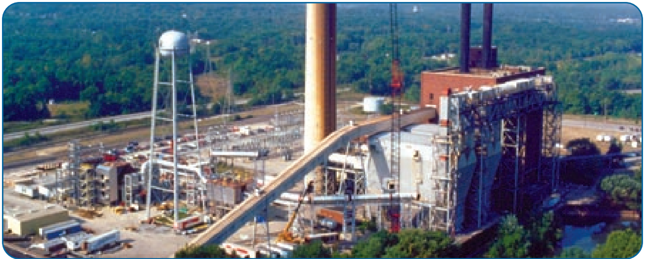
SNOX™ system at Niles Station
