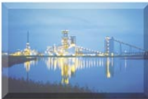
The Tampa Electric Polk Power Station, operating since 1996, is the second commercial U.S. IGCC plant built as part of the DOE Clean Coal Technology Program. It has been in operation commercially since 2001, after completion of its demonstration period under the DOE program. The Polk station generates 250 megawatts of electricity using Texaco/GE gasification technology.
