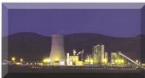
The Puertollano IGCC power plant in Spain is the world's largest coal-based IGCC plant at 330 megawatts capacity. It is owned and operated by the ten-company ELCOGAS consortium. The plant employs the Uhde Prenflo technology to gasify a mixture of coal and petroleum coke feedstock.
