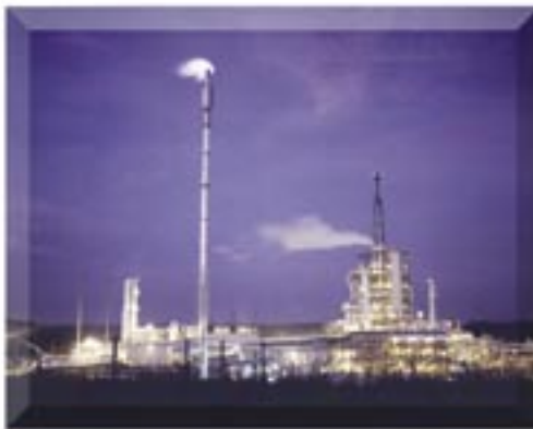
The 262 megawatt Wabash River Repowering integrated gasification combined-cycle (IGCC) plant in Terre Haute, Indiana has been operating since 1995, initially as part of the DOE Clean Coal Technology Program. Using E-Gas technology, the plant has operated more than 15,000 hours, using both coal and petroleum coke feed during its demonstration stage. It is now operating commercially.
