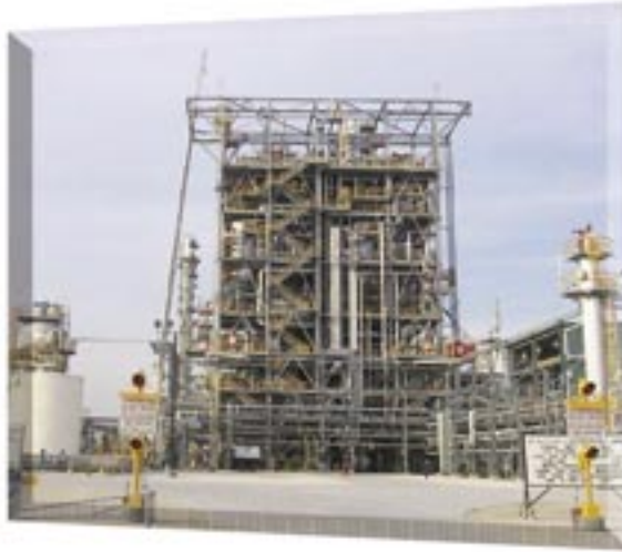
The ExxonMobil Baytown Syngas Plant in Texas is a 240 MW facility that began operation in 2000. Petcoke is used as the feedstock for two GE Energy gasifiers at the plant, which produces both electricity and gaseous fuels.
