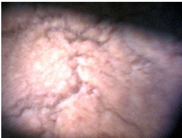
Fig. 5-a Dust cake at bed surface interface viewed through borescope.
