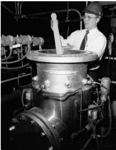
Top of filter vessel and typical filter element
