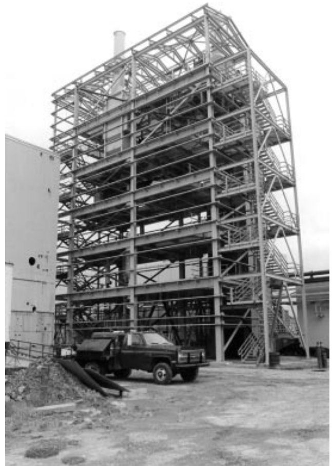
The PDU being constructed at METC
