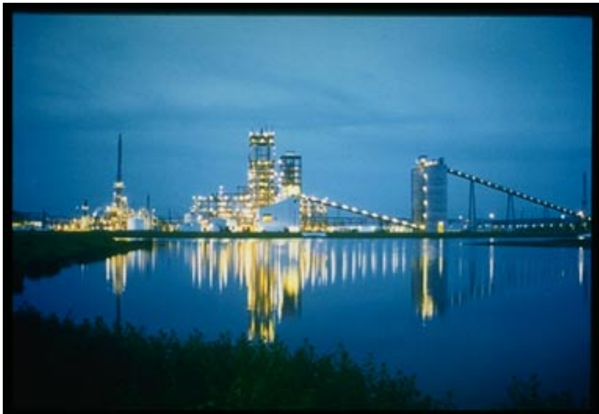
Tampa Electric Co. IGCC Polk Power Station
