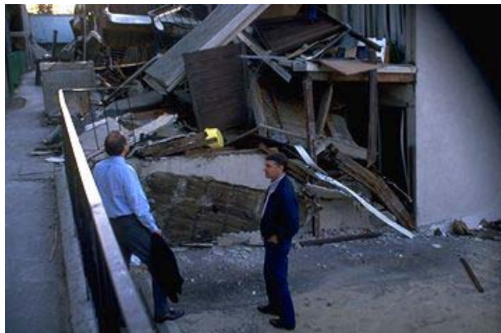
Northridge Earthquake, CA, January 17, 1994 -- Buildings, cars and personal property were all destroyed when the earthquake struck. Hundreds of thousands of residential and commercial structures were damaged and 72 deaths were attributed to the earthquake. Damage costs were estimated at $40 billion. (Photo obtained from FEMA's photo library.)
