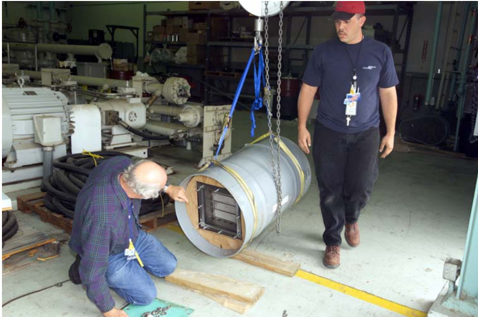
Figure 8. Packaging Preparation. Pellet Tray Removal (I), Bldg. 836B From left, Bruce Clegg (LLNL) and Rich Villafana (LLNL)
