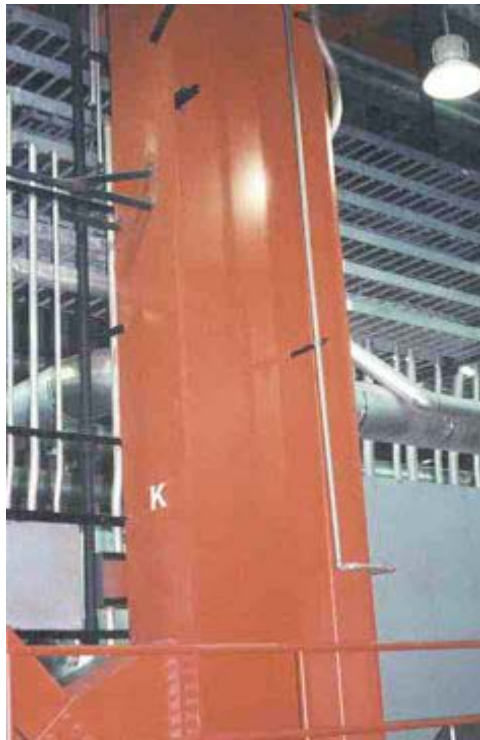
Figure C.4: Example of the Steel Beams in Turbine Hall
