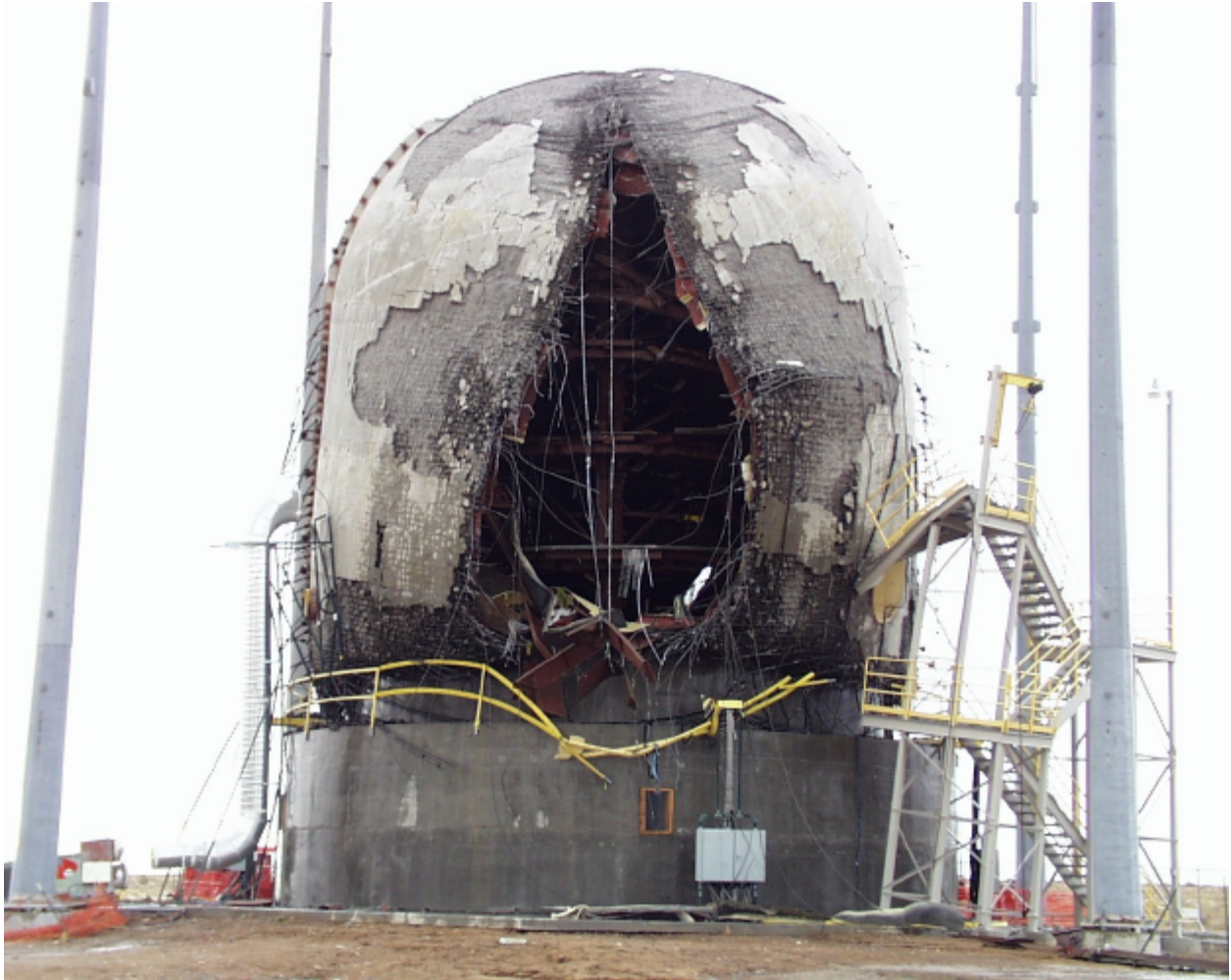
Figure 1-6. PCCV Model after Structural Failure Mode Test
