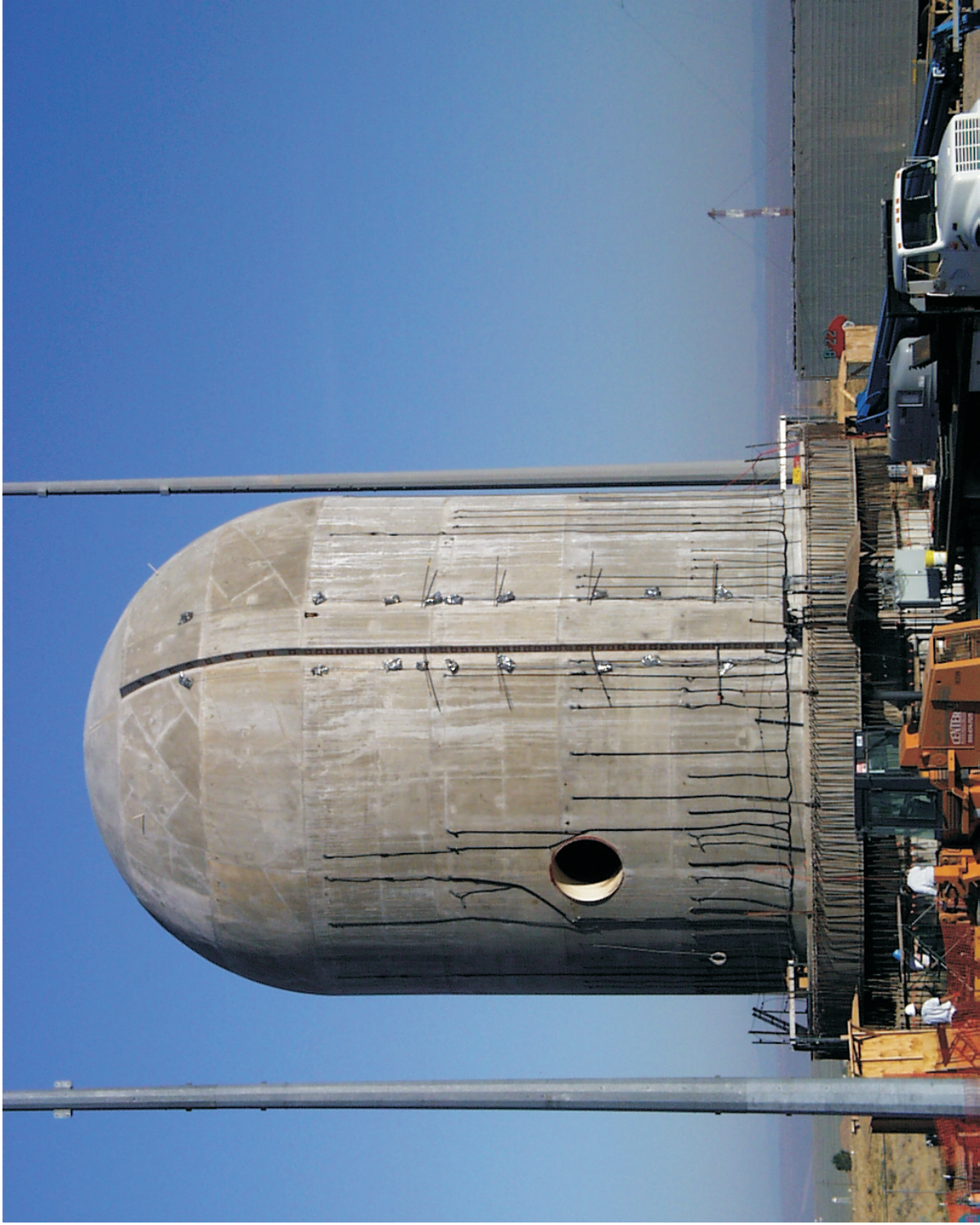
Figure 1-1. NUPEC/NRC 1:4 Scale PCCV Model Built at Sandia National Laboratories
