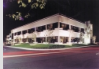
Housed in an 87,000-square-foot facility at Southwest Research Institute, the CNWRA offers sophisticated computational and visualization resources and extensive laboratories to solve diverse scientific and technical problems for government and industry.
