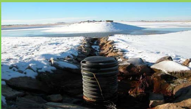
CBNG impoundment operated by J.M. Huber near the Wyoming/Montana boarder.
