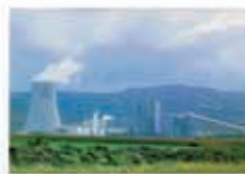
ELCOGAS Power Plant; Puertollano, Spain
