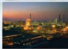
Sasol Synfuels Plant; Secunda, South Africa
