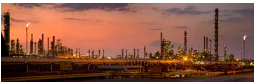
Gasification has been important since the mid 1950s in South Africa when the original plant was built using fixed bed, dry bottom gasifiers.
