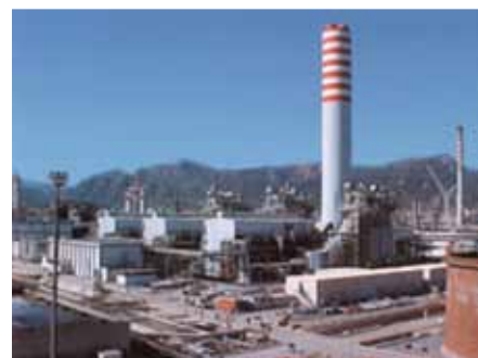
The Sarlux IGCC at the Saras oil refinery in Sardinia is the largest operating IGCC to date, producing 550 MW of electric power. The plant also co-produces hydrogen and process steam from visbreaker tar. The plant completed start-up in 2000.
