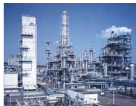
The Nippon Petroleum Refining Company Negishi IGCC plant began operations in 2003. This is the first IGCC plant in Japan and gasifies 2,000 metric tons per day from the Negishi refinery in Yokohama.
