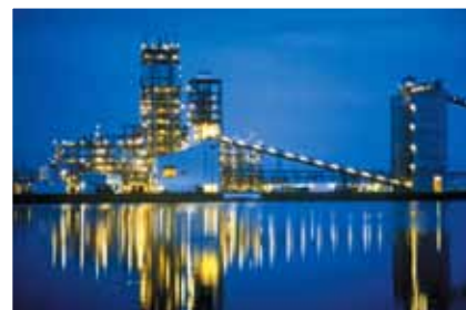
Tampa Electric Polk Power Station
