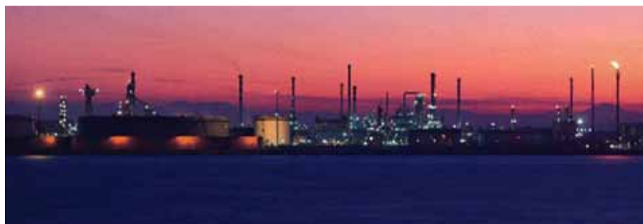
The Shell Pernis Refinery in Rotterdam uses the Shell Gasification Process to convert heavy refining residues into hydrogen for a hydrocracker as well as syngas for power generation. Three gasifiers process 1,650 tons per day of residues. First started in 1997, it has accumulated approximately 40,000 hours on syngas. This 115 MW IGCC plant automatically switches to backup fuels to maintain high reliability of the hydrogen and steam.
