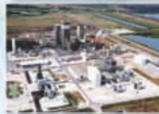
Tampa Electric Polk Power Station; Florida, United States
