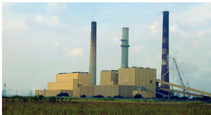
Ghent Power Station
