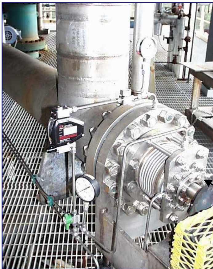
Figure 3.5-4 Inlet-Side Seal Packing Follower (Eight-Bolt)
