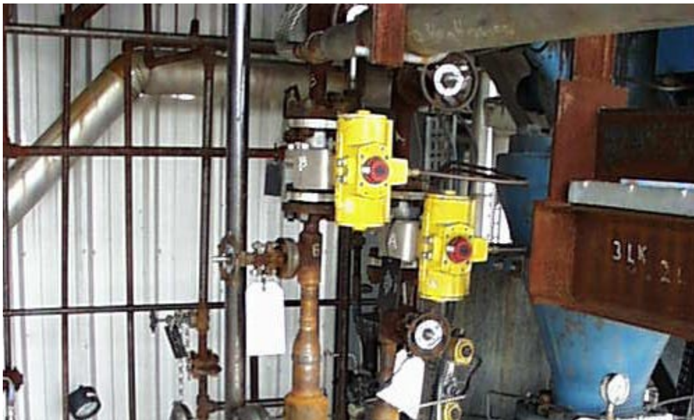
Figure 3.5-2 FD0520 Vent Line Addition
