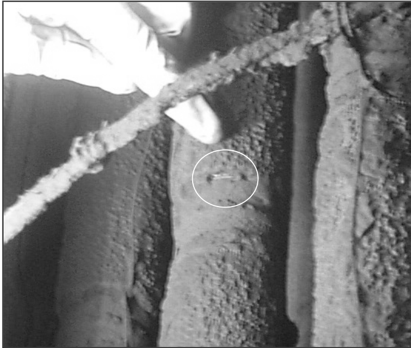
Figure 3.3-10 Potential Leak Path on Fairey Microfiltrex Metal Element (B35)
