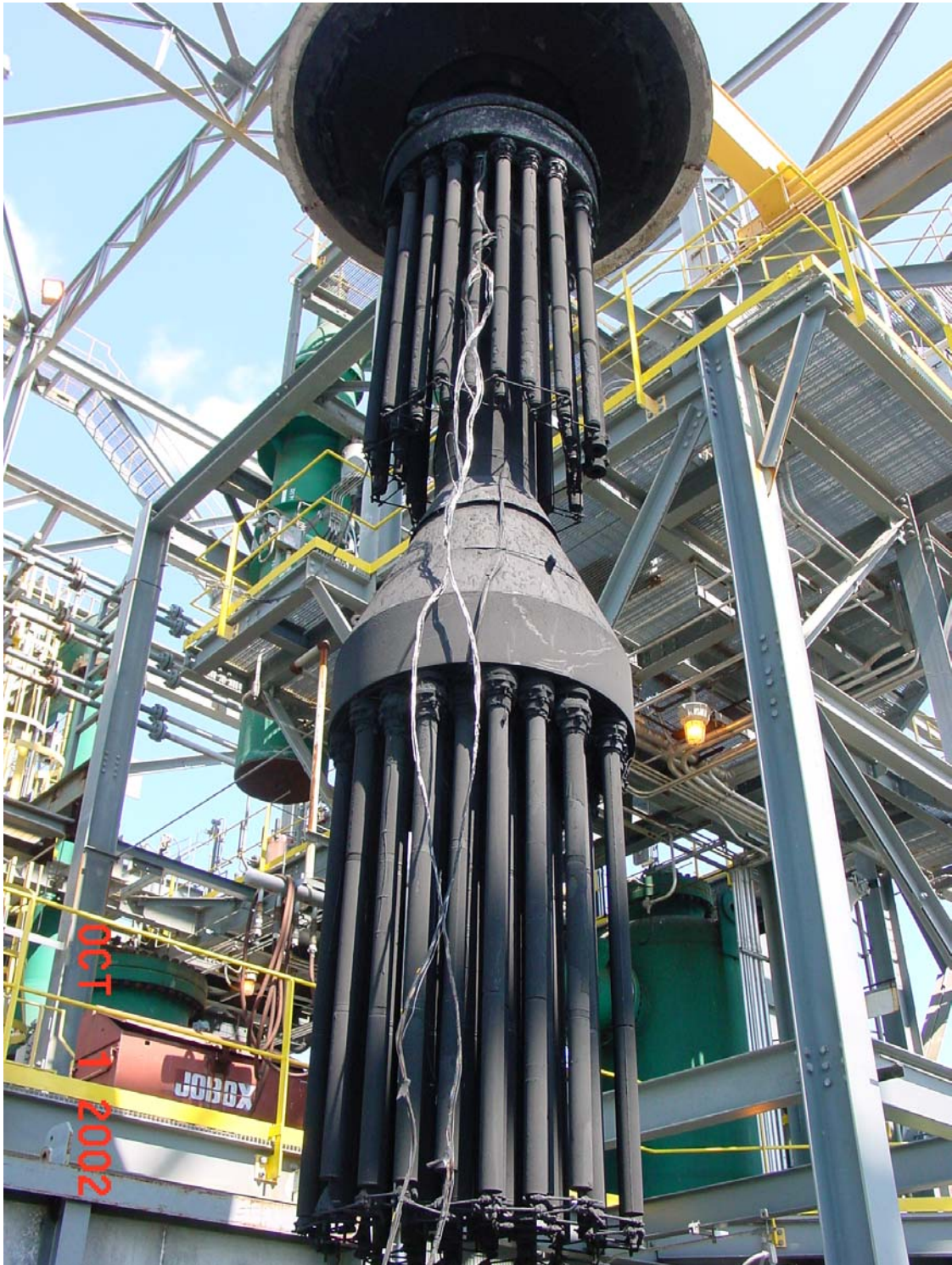
Figure 3.3-4 Tubesheet Removal After TC09
