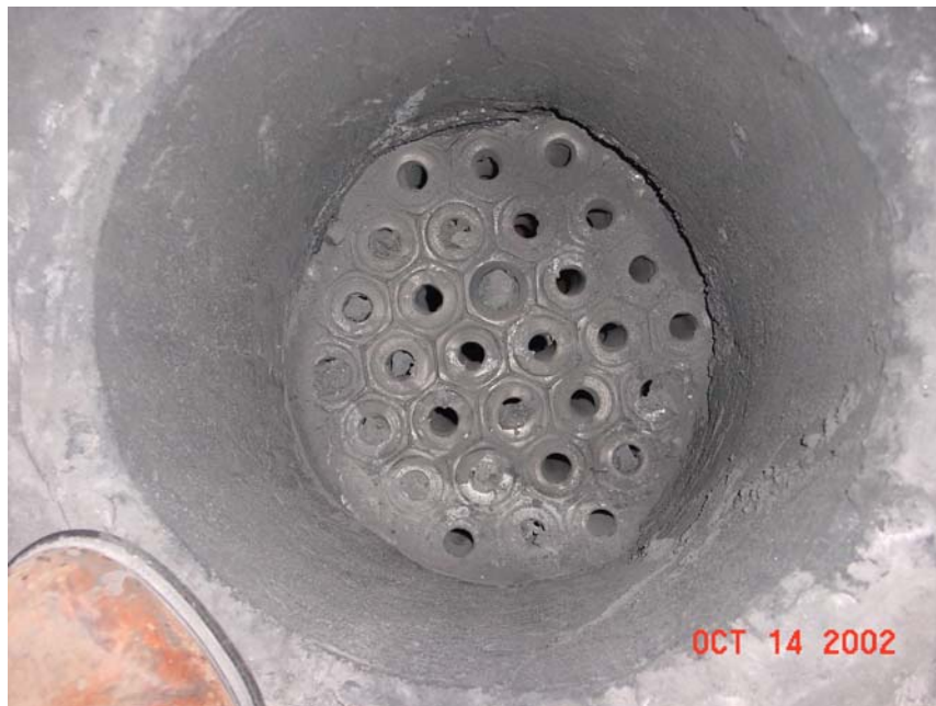
Figure 4.1-9 HX0202 Tube Sheet
