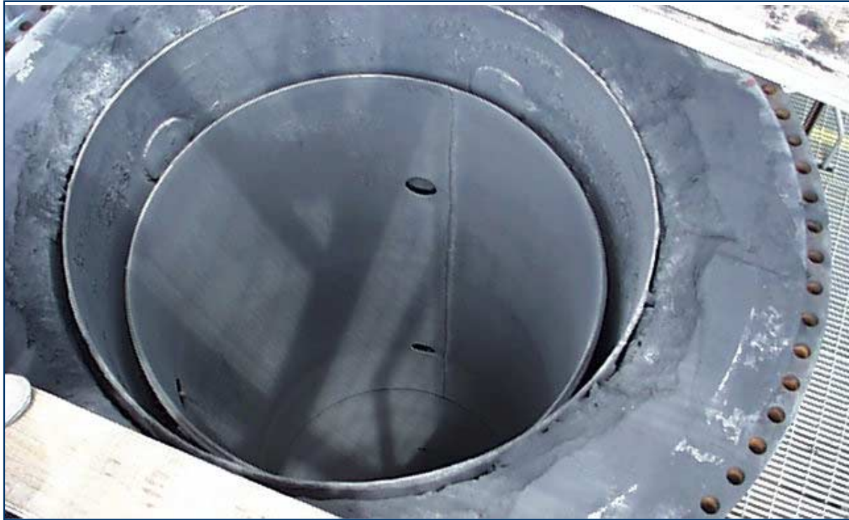
Figure 3.3-8 Char Accumulation on Shroud and Liner Sections
