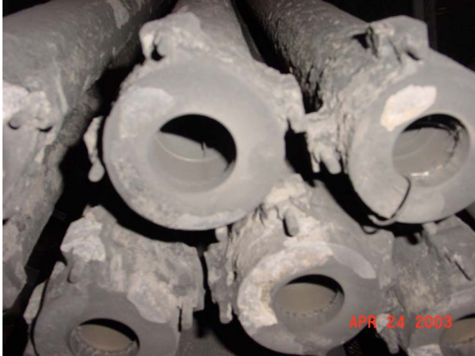
Figure 4.3-9 Inverted Filter Assembly After TC11
