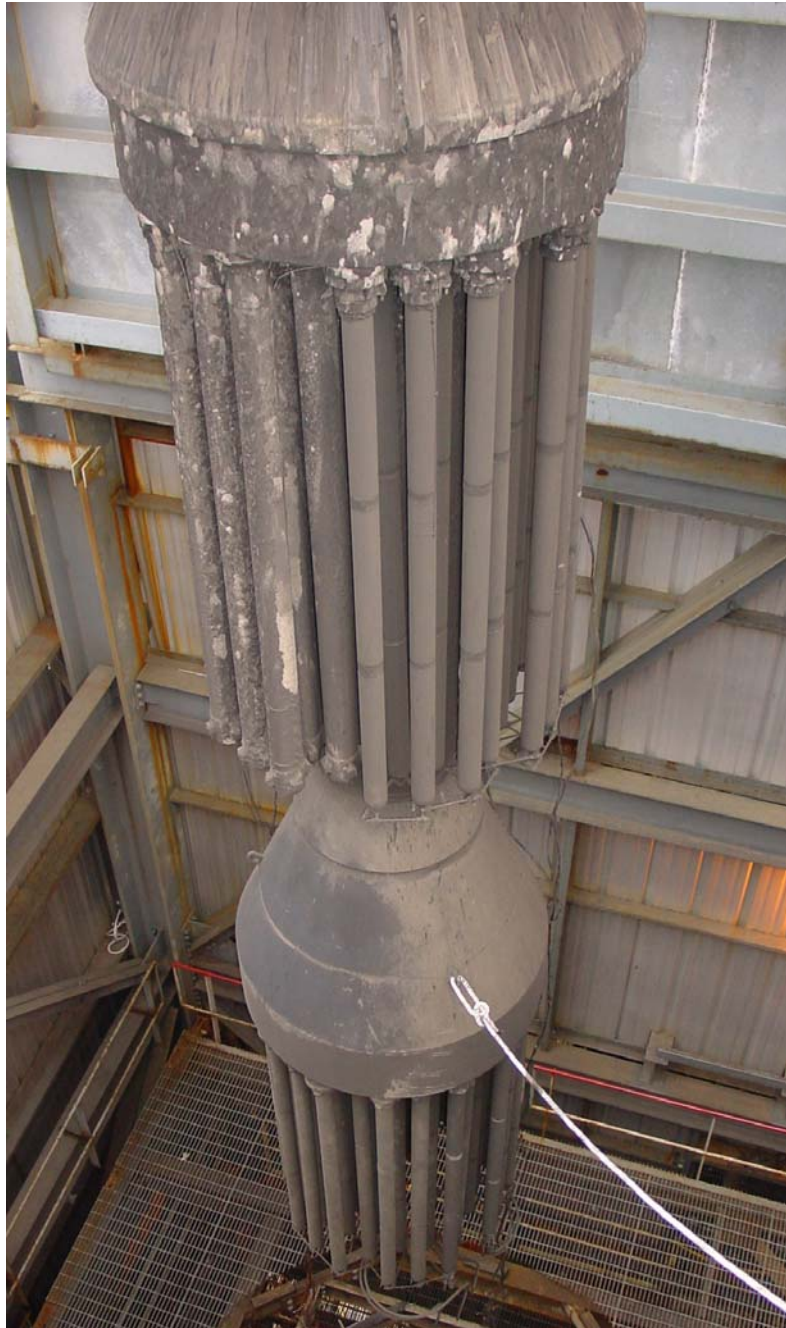
Figure 4.3-2 PCD Plenum Removal After TC11
