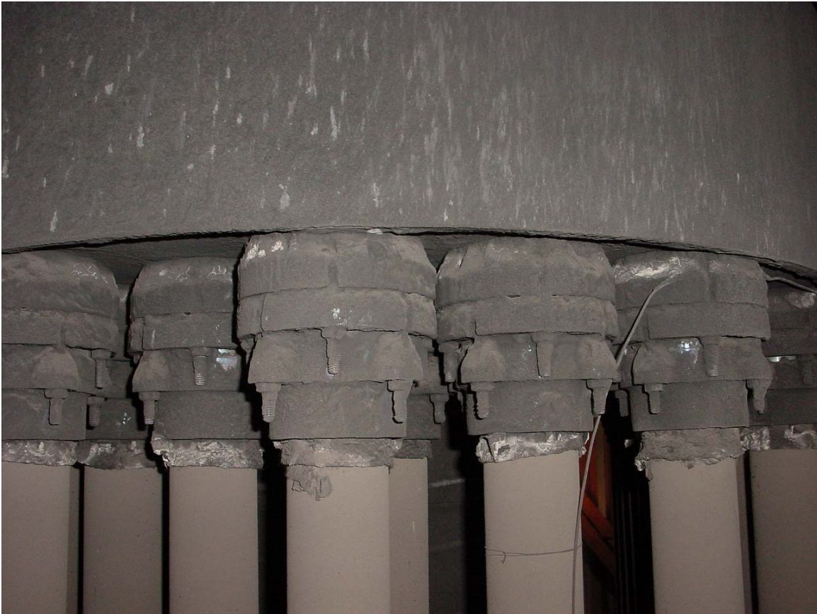
Figure 3.3-13 G-ash Build-Up on Filter Holders After TC07D
