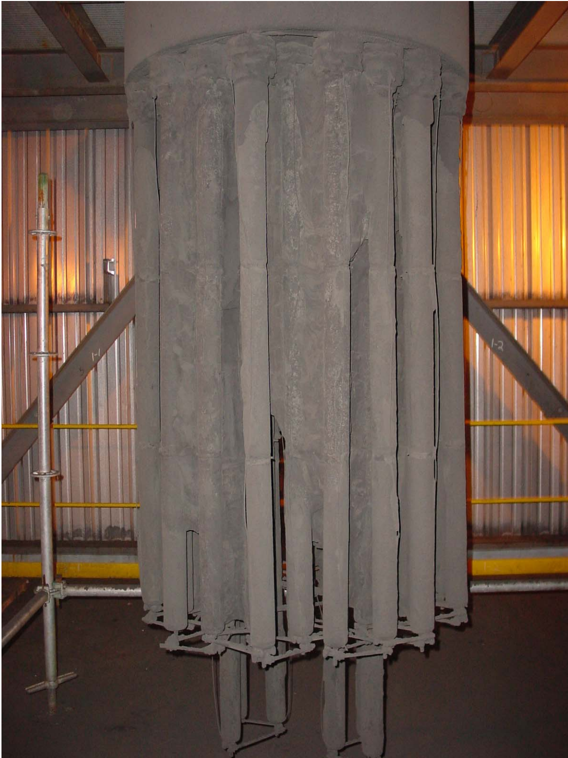
Figure 3.3-2 Char Bridging on FL0301 Bottom Plenum
