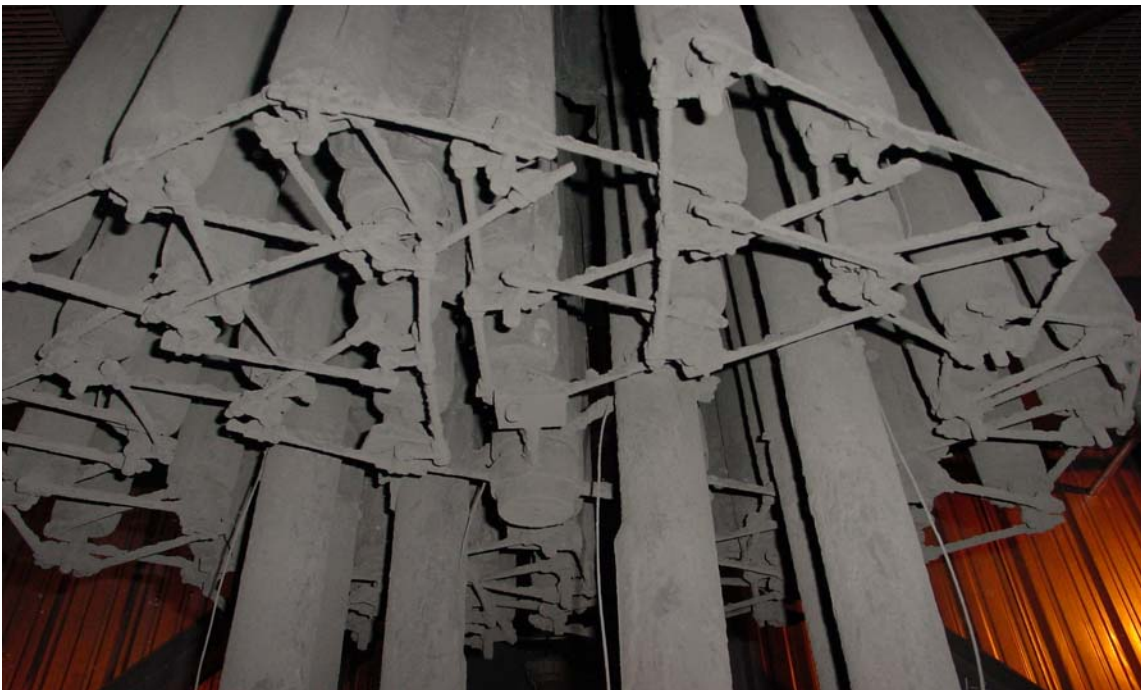
Figure 3.3-4 Char Build-up on Bottom Plenum Support Brackets
