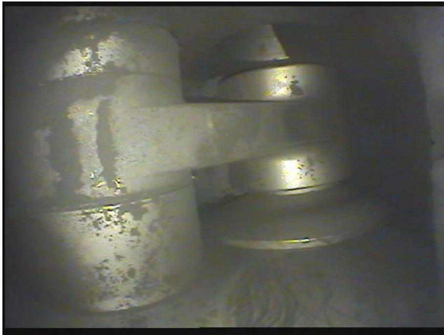
Figure 4.3-13 Everlasting Valve Rotating Disc Valve
