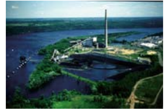
Large Electric Power Generating Plants
