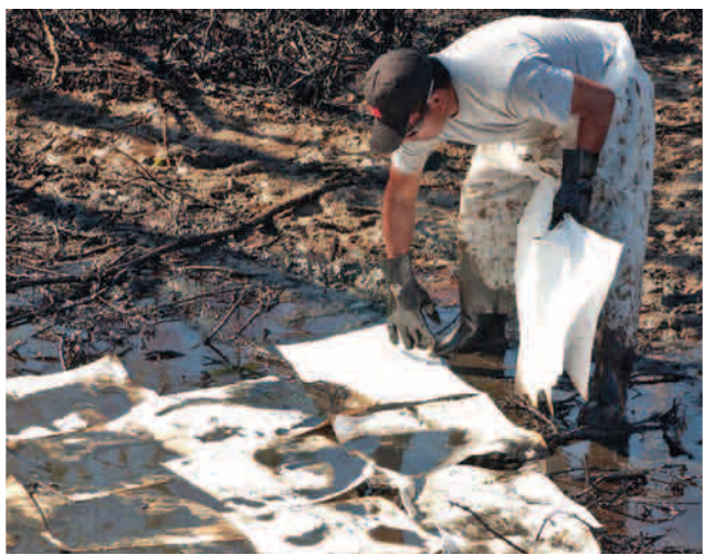
A slicker picker-upper. Absorbent pads are used to clean up surface oil at the Bass Enterprises South Facility in Cox Bay, Louisiana, where Katrina caused the release of an estimated 3.8 million gallons of oil. Oil spills may have long-lasting effects on water supplies and surrounding ecologies.
