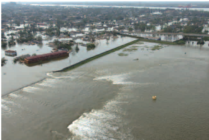
Hope for renewal. Use of innovative construction and maintenance technologies may allow engineers to rebuild the New Orleans levee system (shown here flooding the Ninth Ward on 30 August 2005) stronger than before.
