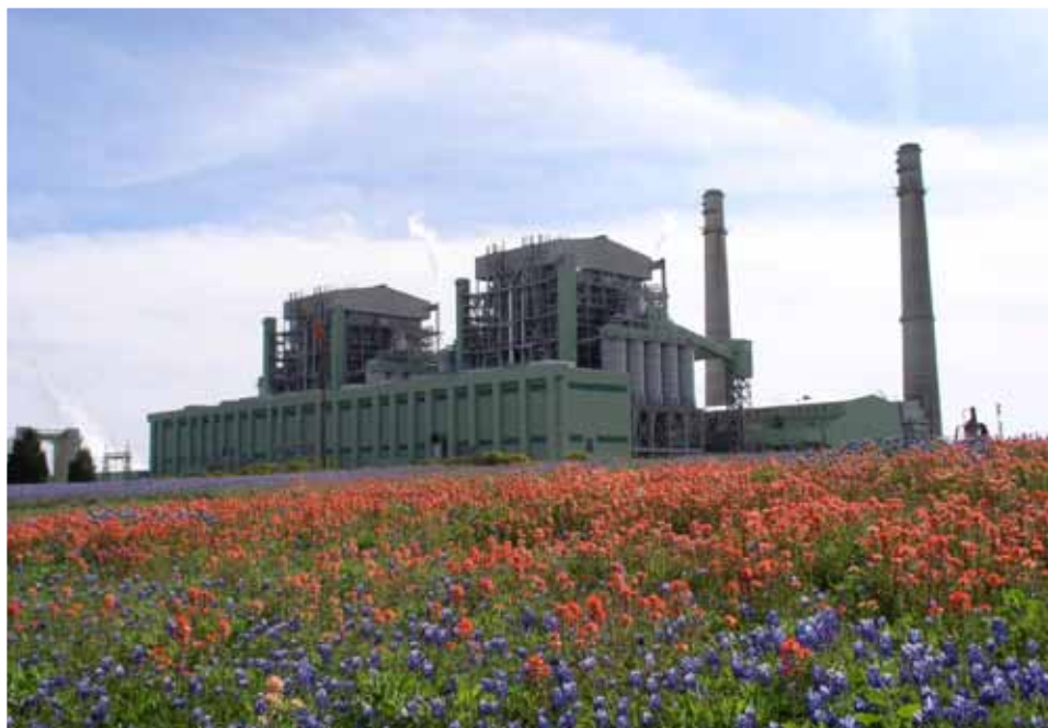
NRG Texas's Limestone Power Plant in Jewett, Texas
