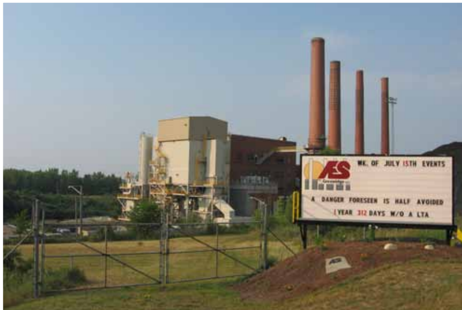
View of AES Greenidge Showing Demonstration Facility
