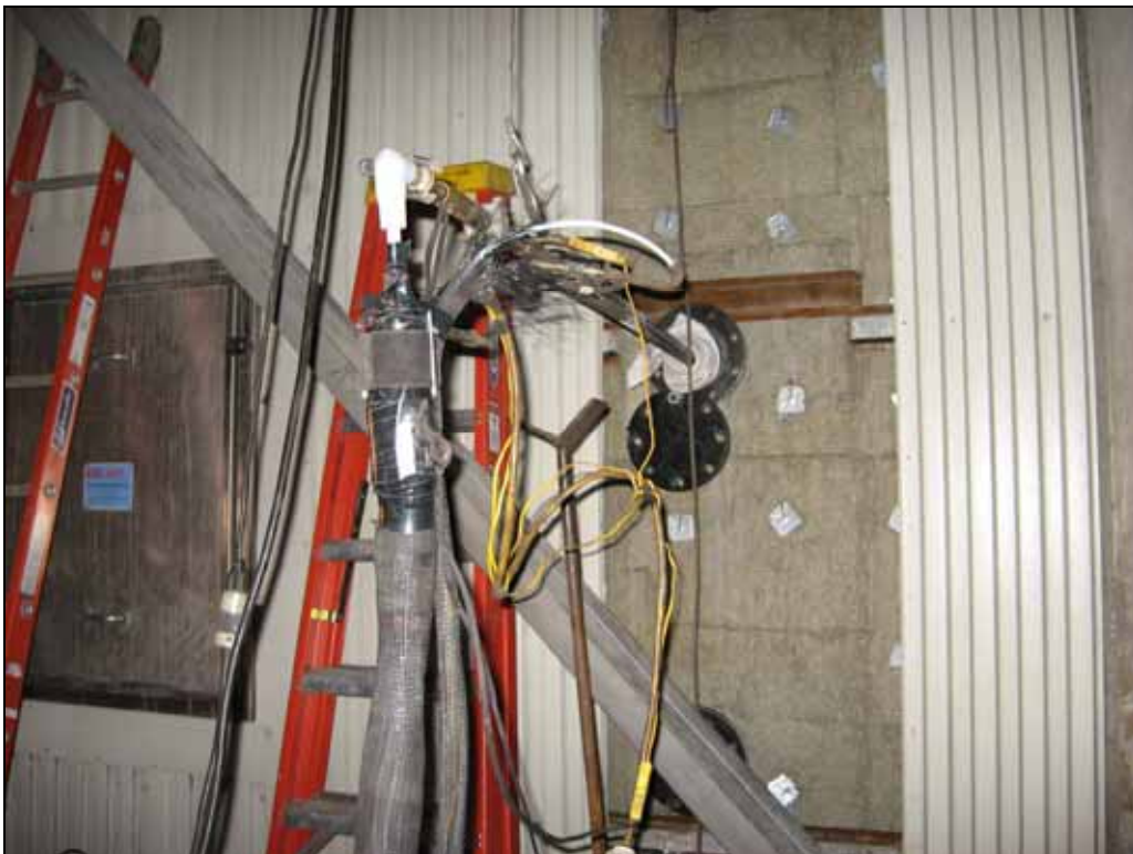
Figure 5. Photograph of flue gas Hg sampling at the air heater outlet.
