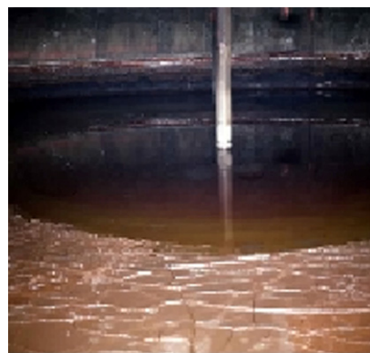
Figure 1: At the Hanford site, 53 million gallons of high-level radioactive and chemical waste are stored in 177 underground tanks.
