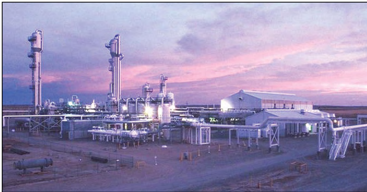
Figure 6. Enterprise Natural Gas Processing Plant
