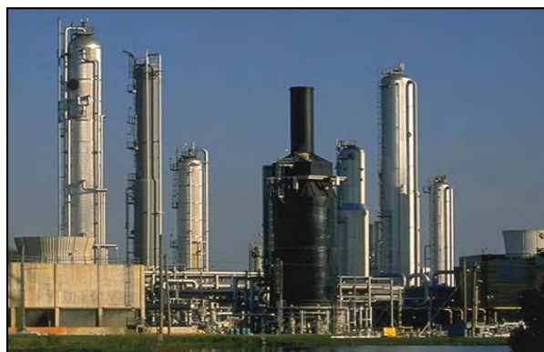
Figure 7. Promix Fractional Plant
