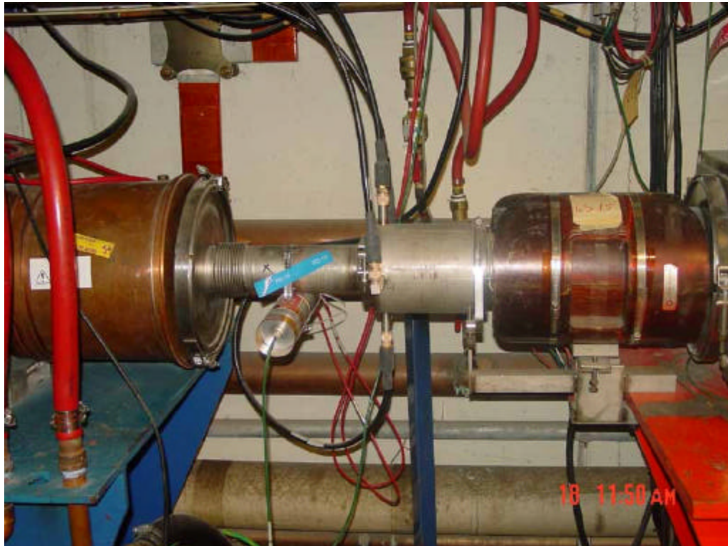
Booster Water Tube Replacement
