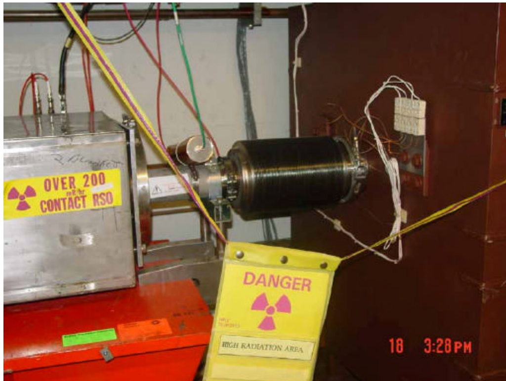
Beam Positioning Monitor Replacement in Long 6
