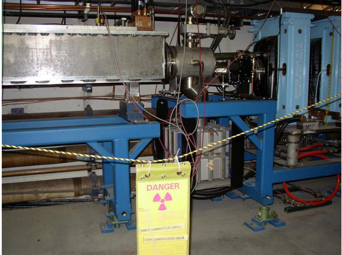
MP01 Long 13 Magnet Replacement
