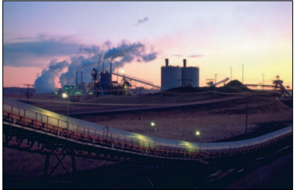
ACCP facility during construction.
