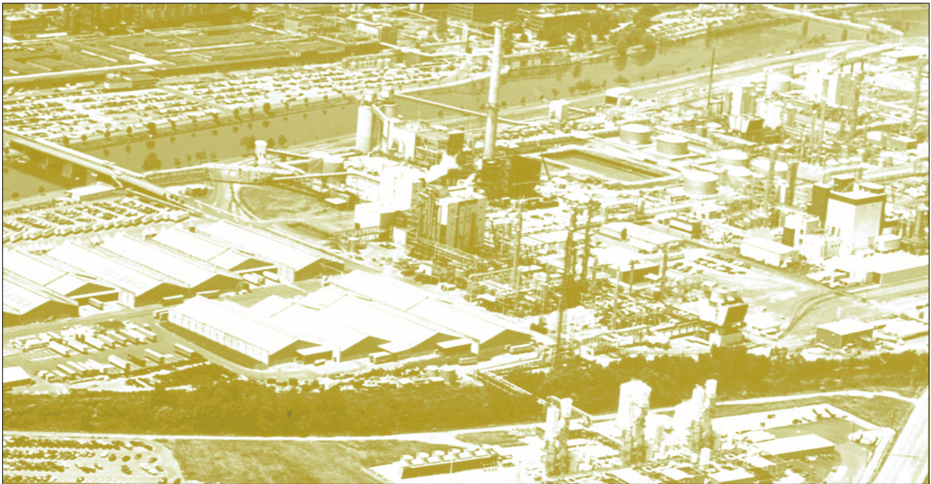
Eastman Chemical Company's chemicals-from-coal complex at Kingsport, Tennessee
