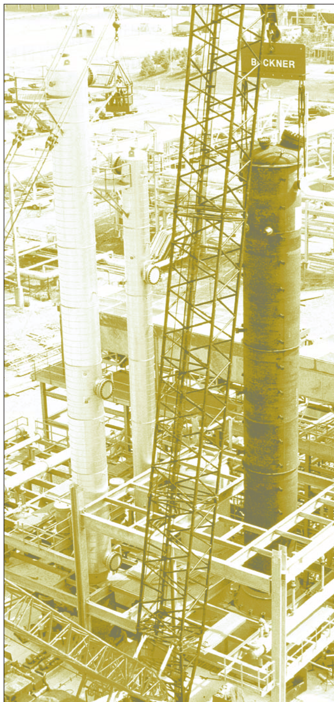
SBCR being installed
