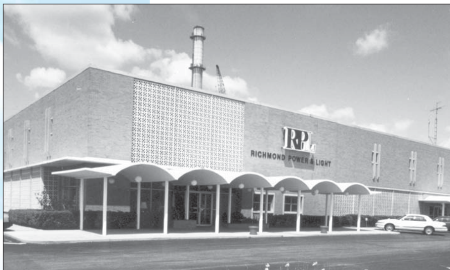
Entrance to Richmond Power and Light Company's Whitewater Valley Station
