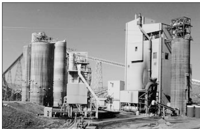
Process unit enclosure with PDF silo on right and coal storage silos and train loading station on left
