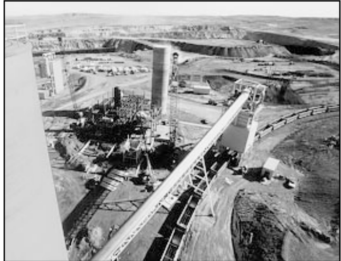
Loading out coal train from coal bunker
