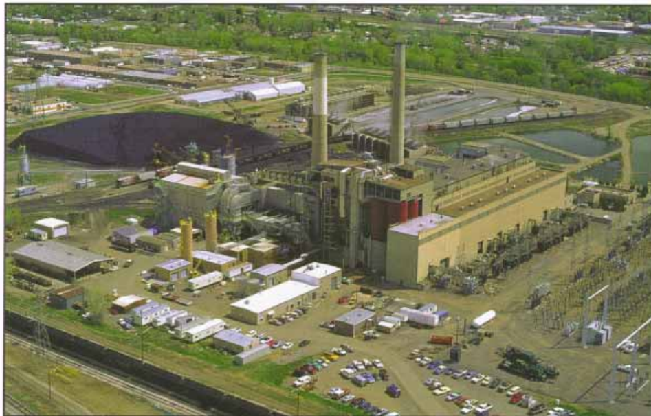
Public Service Company of Colorado's Arapahoe Station, site of a vertically fired boiler project designed to demonstrate LNB+OFA technology for NO x reduction.
