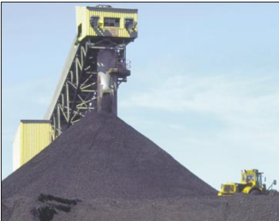
Coal unloading facility.
