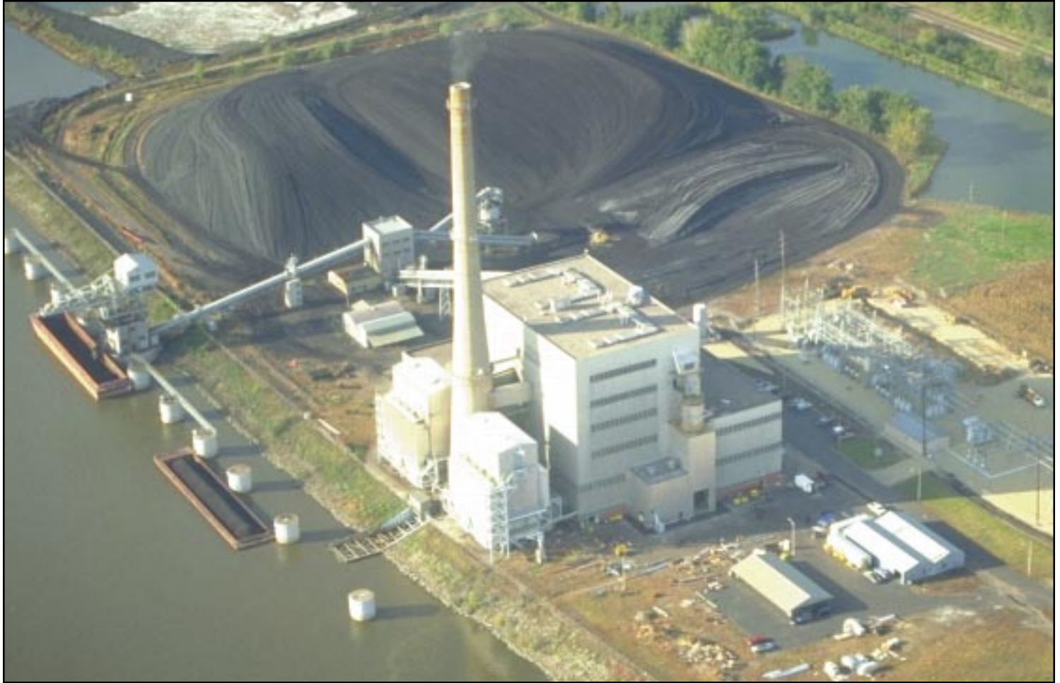
Aerial view of Nelson Dewey Station.
