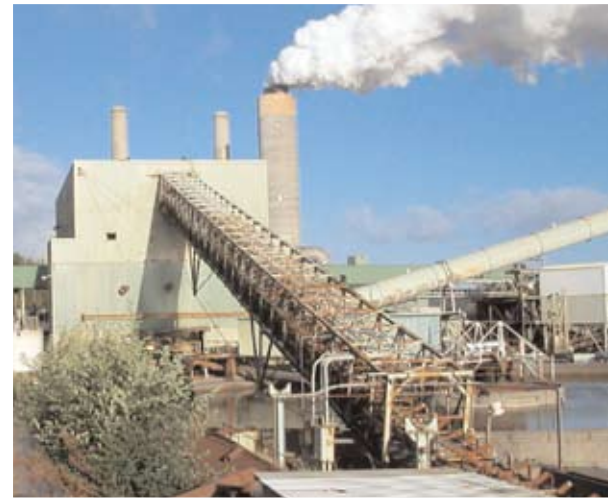
TransAlta's 1400 MW coal-fired power plant in Centralia, Washington.
