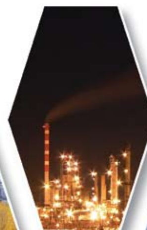
Gas Processing Plant
