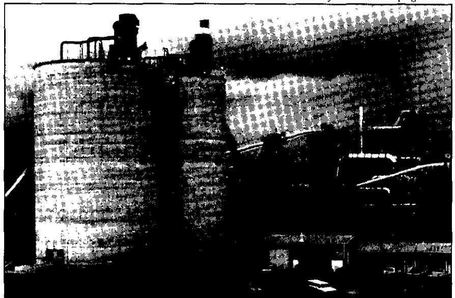
Rosebud SynCoal™ 1,000 tons-per-day advanced coal upgrading facility located in Colstrip, MT.
