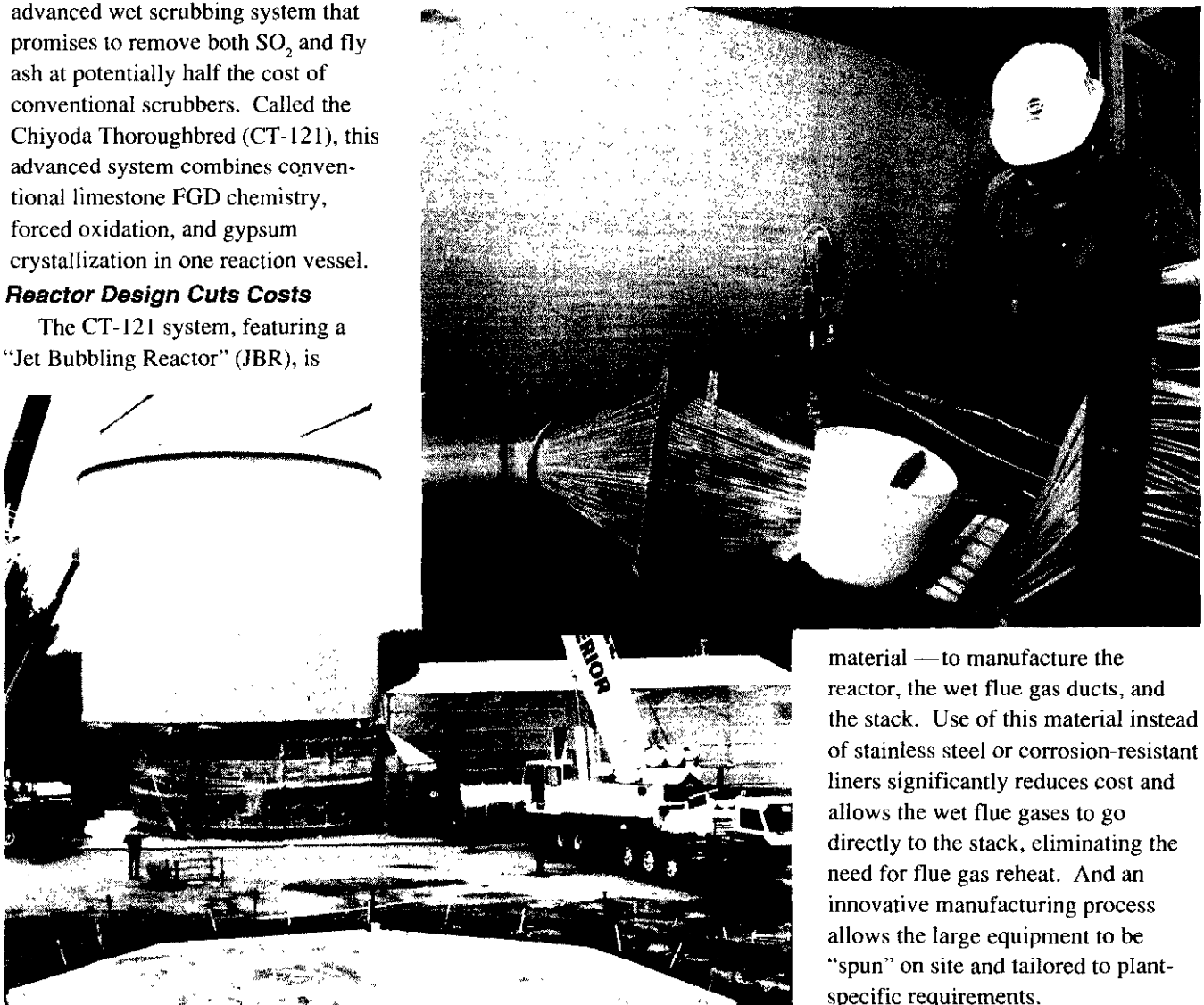
Right: A unique spinning process was used to fabricate the reactor shell on site in less than 30 days. Above: The completed vessel being lifted from the mold for placement onto the foundation.
