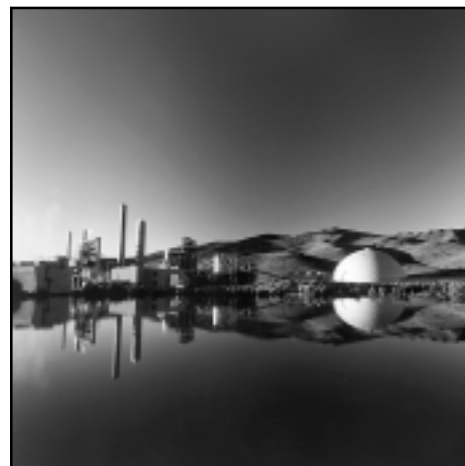
SPPC's Piñon Pine project demonstrates air-blown, fluidized-bed IGCC technology using hot gas cleanup, and evaluates a low-Btu gas combustion turbine.
