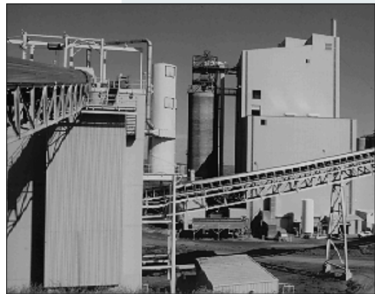
The ENCOAL® project demonstrates the integrated operation of a number of processing steps to produce two higher value fuel forms from mild gasification of low-sulfur subbituminous coal.
