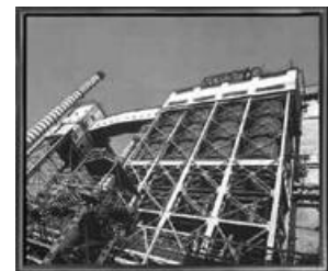
Power plant in Korba, India
