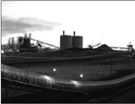
ACCP Raw Coal Handling System (in foreground).
