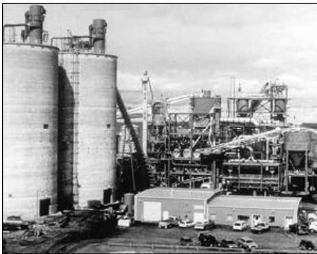
ACCP storage silos.
