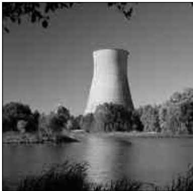
Shown above, a typical power plant cooling tower
