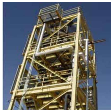
Process Development Unit at WRI Advanced Technology Center
