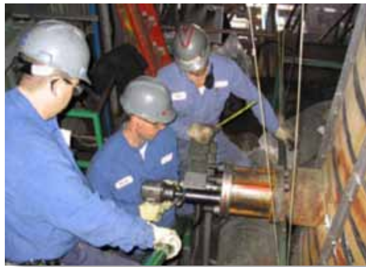
Test thermocouples being installed in a commercial gasifier
